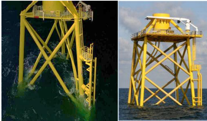
Figure 1-11: Jackets à 3 jambes [The Northern Times, 2020] et à 4 jambes [University of Strathclyde, 2014]
